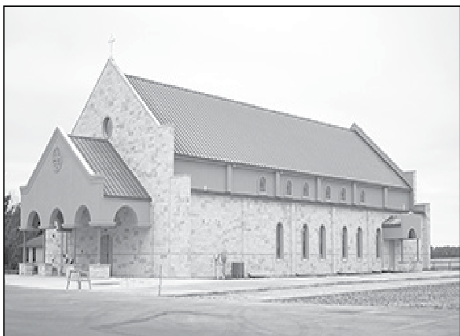
Saint Stephen Catholic Church Building complete and ready for dedication
