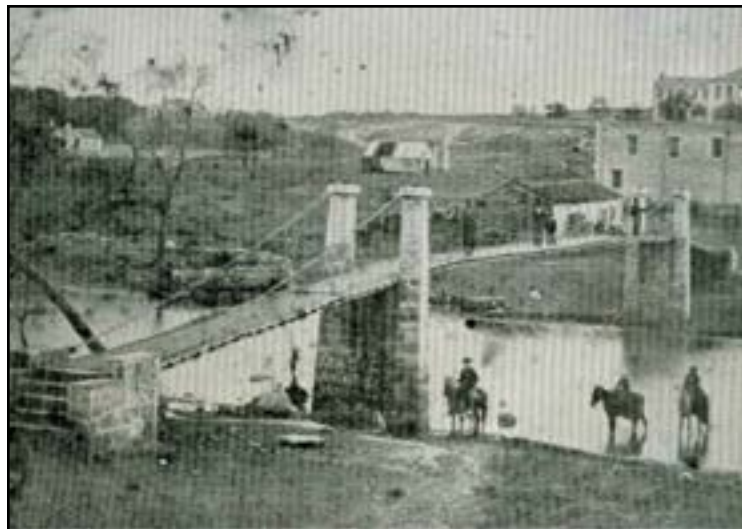
This photo, courtesy of the Salado Historical Society, shows the walking bridge over Salado Creek. In the background is Salado College.
