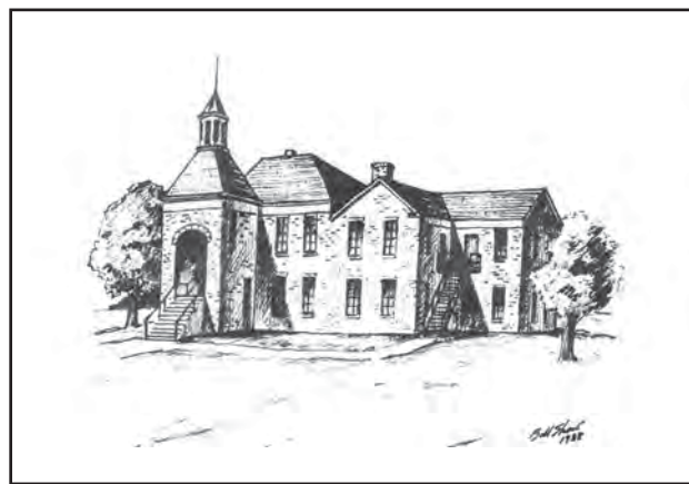
The original structure of the college building was the ell shaped structure to the right. The college chapel was located on first floor on the far right side of the building.
