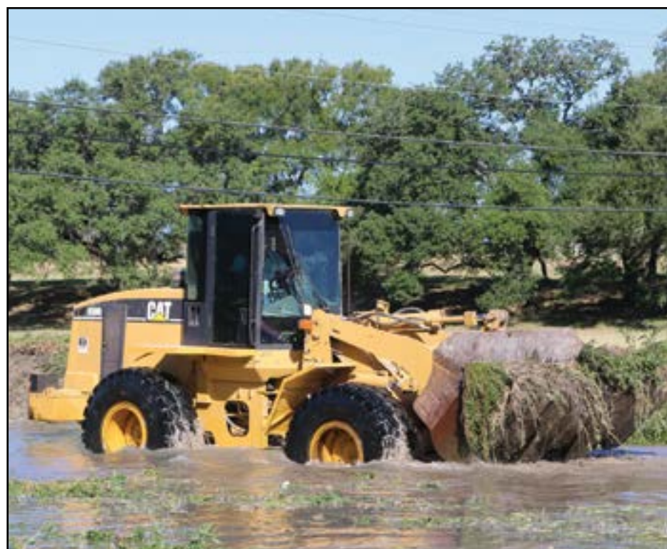
Lone Star Grading and Paving removed about 1,000 tons of gravel and debris that has collected over the past few years at the low water crossing of Salado Creek in Mill Creek. The work was completed under a permit from Texas Parks and Wildlife. (PHOTO BY MARILYN FLEISCHER)
