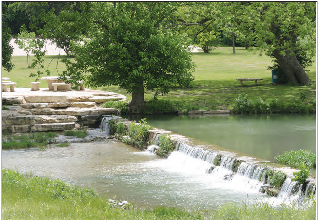
It's been several years since the water flowed over the Stagecoach Dam like this, an indication that the area has finally moved out of the prolonged drought. (PHOTO BY ROYCE WIGGIN)
