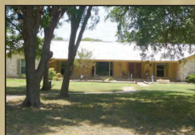
2289 Sulphur Wells Rd. on 7.7 ac., Belton $529,021
