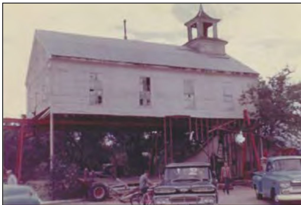
For 80 years, the Salado Masonic Lodge was the second story of the First Baptist Church of Salado sanctuary, built in 1878. The Baptists and Masons shared title to the two-story building with the Baptist Church meeting downstairs and the Masonic Lodge meeting upstairs. In 1958 when the Baptist Church built a new all-brick sanctuary building, the Masonic Lodge moved the second floor to its home on Church Street on a lot donated by Charlton Johnson, a Past Master of Salado Lodge. The humble frame building has served as the home of Salado Masons for 139 years.
