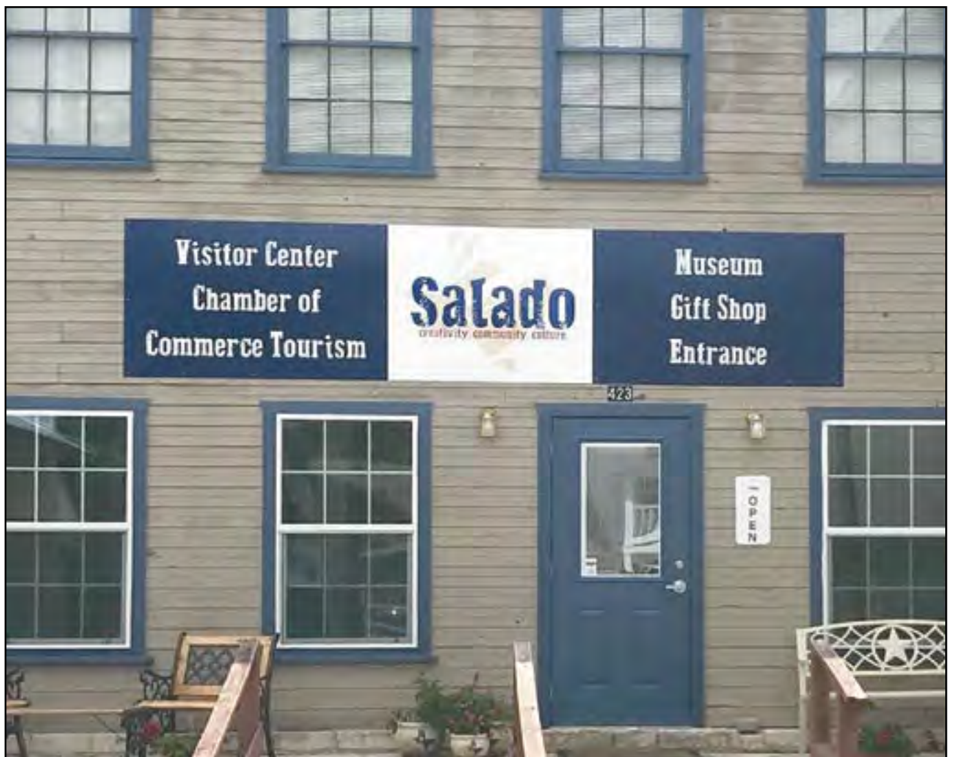
The Salado Chamber of Commerce and Tourism Bureau will hold an Open House for the new Visitors Center and Chamber offices at 423 S. Main St. in Salado. The open house will be 11 a.m.-3 p.m. June 15. Everyone is invited to visit the newly renovated Visitor Center, the Chamber/Tourism offices, the Wee Scots Shop, and the Salado Museum. Come take a tour and visit with staff. (PHOTO COURTESY SALADO CHAMBER OF COMMERCE)
