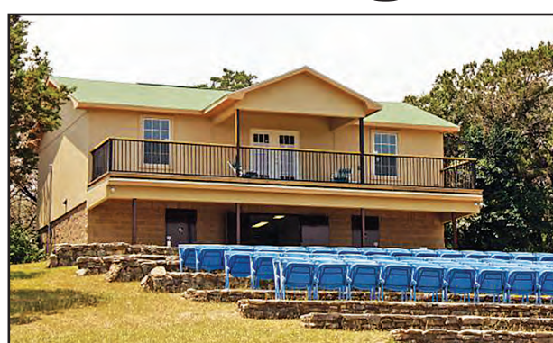
The new building at Tablerock will serve as a refreshment center, restrooms and an upstairs room for education purposes, including the annual Summer Camp.
