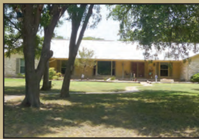
2289 Sulphur Wells Rd. on 7.7 ac., Belton $529,021
