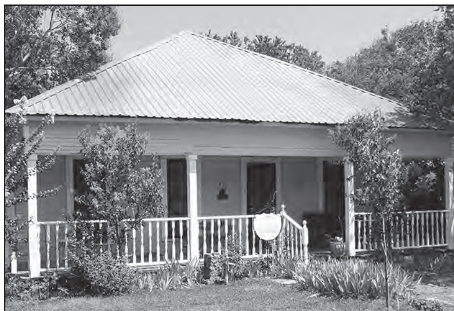
The Norwood House on Main Street.
