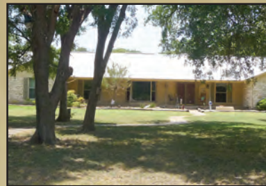
2289 Sulphur Wells Rd. on 7.7 ac., Belton $529,021
