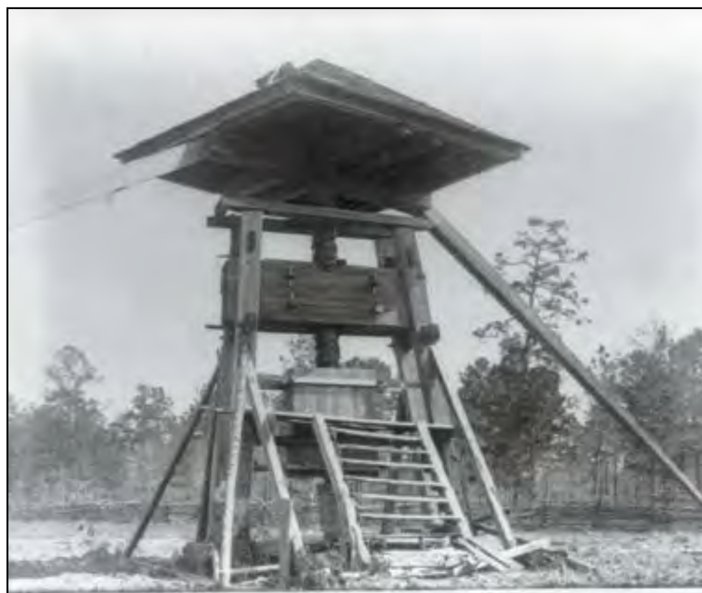
Wooden screw press used for making cotton bales. (PHOTO LIBRARY OF CONGRESS LC-USZ62-30090.)
