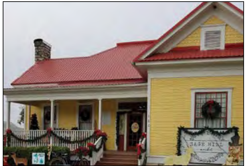
Not much of the Vickrey influence on the Vickrey-Berry House can be seen today.
