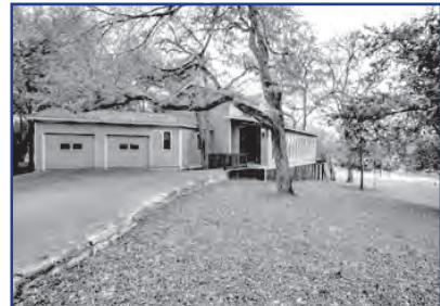
128 ROCK CREEK DRIVE
