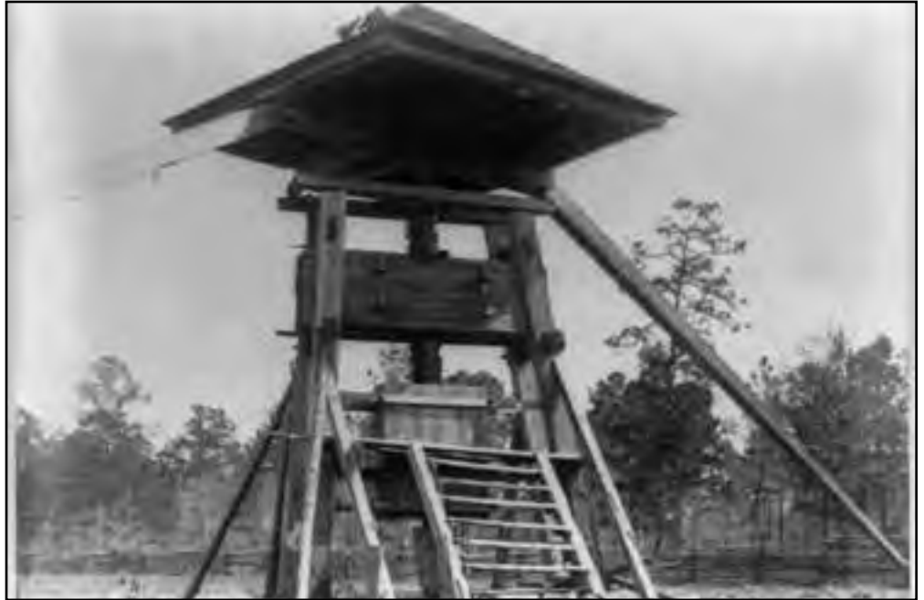
Wooden screw press used for making cotton bales. (Library of Congress LC-USZ62-30090.)
