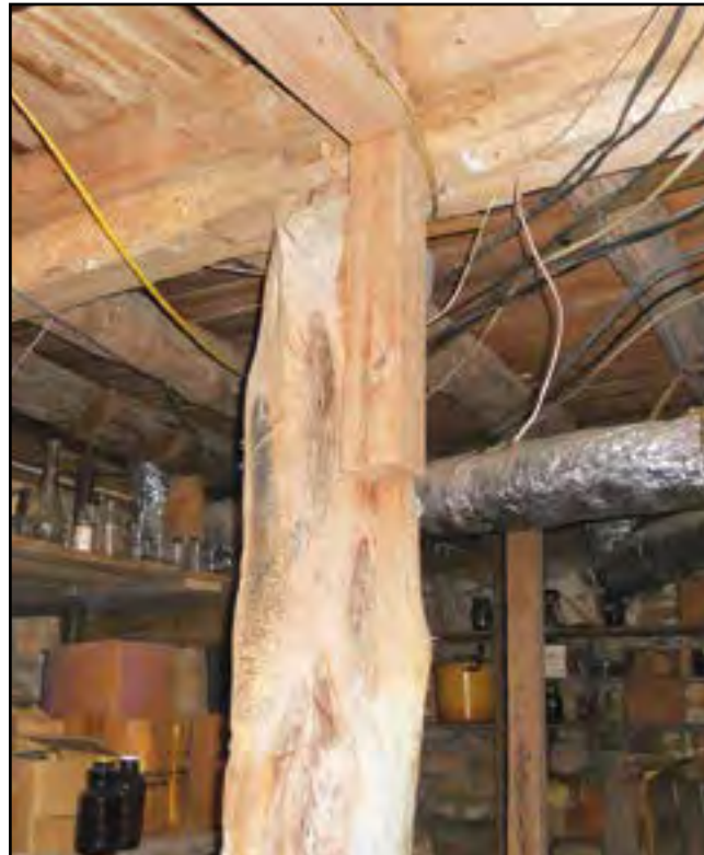
Solid cedar beams and a limestone foundation have stood the test of time as the Anderson House has been on South Main Street since 1860. (PHOTO COURTESY KINNISON FAMILY)
