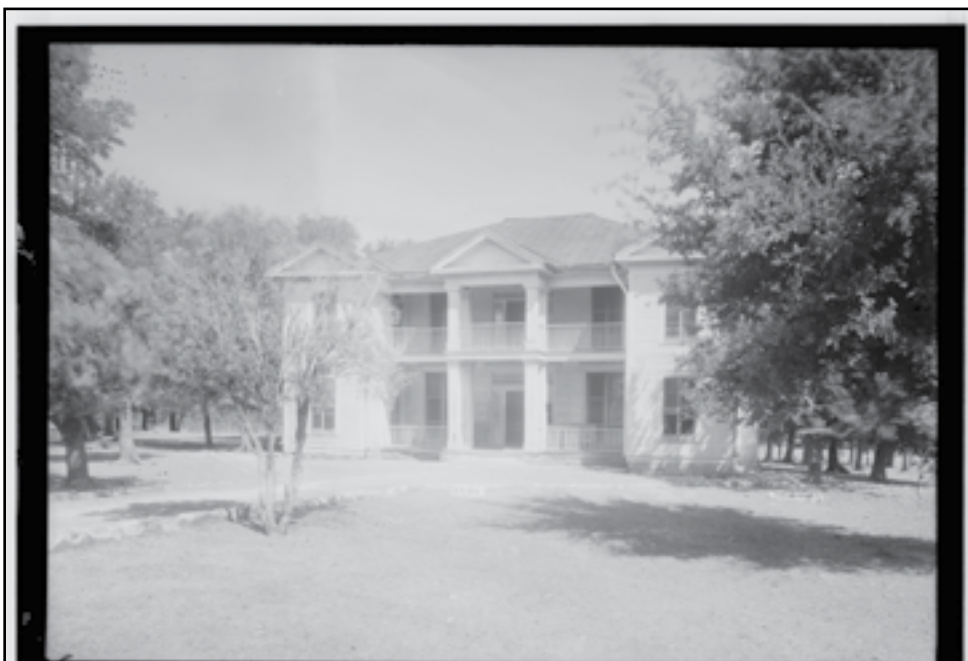
Historic American Buildings Survey, Arthur W. Stewart, Photographer September 11, 1936 SOUTH ELEVATION (FRONT). - E. Sterling C. Robertson Plantation House, West access road, I-35 vicinity, Salado, Bell County, TX PHOTOS FROM SURVEY HABS TX-394 Documentation Compiled After. Photograph. https://www.loc.gov/item/tx0155/ .
