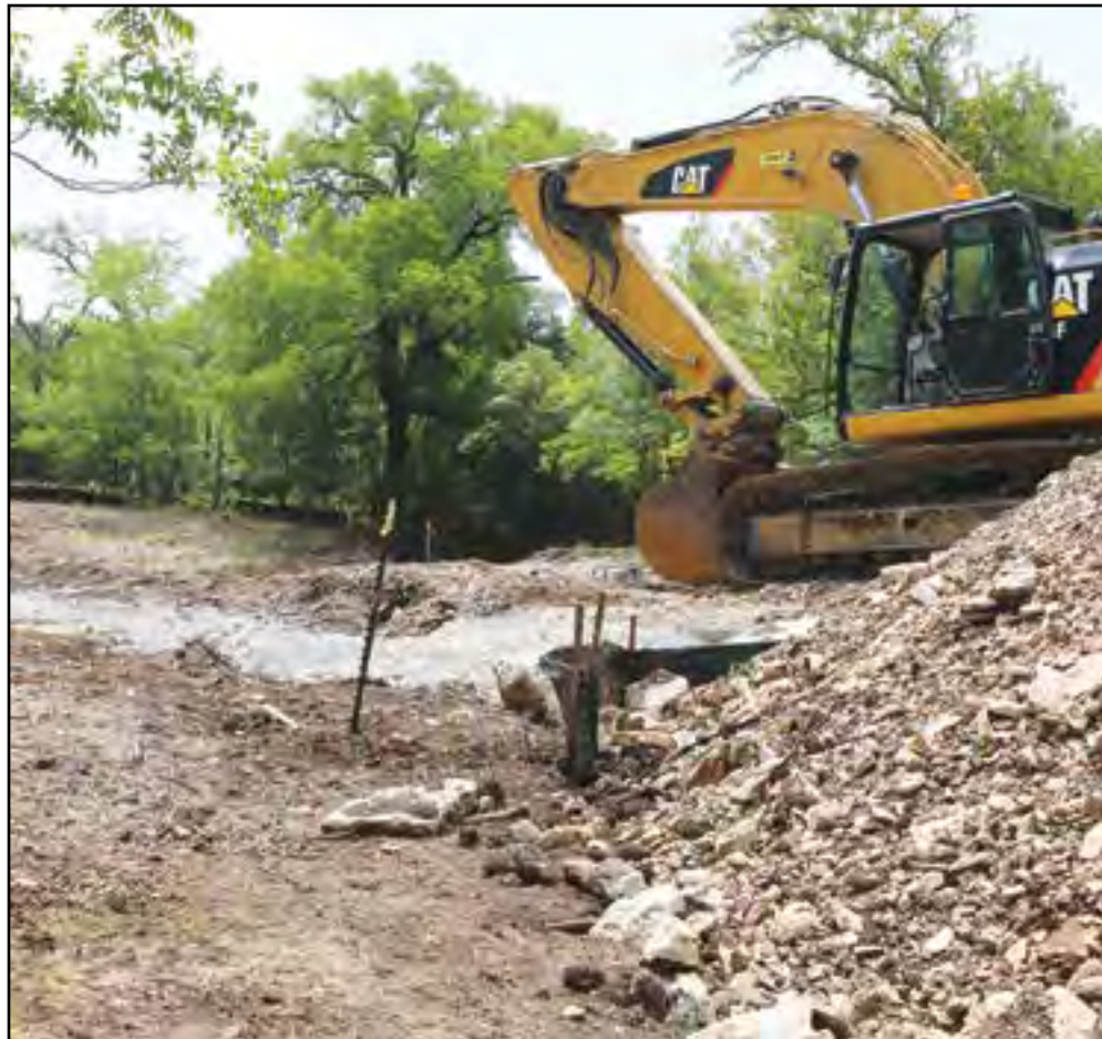
Work crews from James Construction have begun to remove the low water crossing on Rose Lane. The crossing will be replaced with box culvert structure that will pass a 100-year storm event. Work is expected to continue through Oct. 31. (PHOTOS BY ROYCE WIGGIN)
