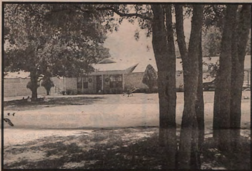
Over 5,000 square foot, office and storage for retail or commercial with beautiful 3 bedroom, 2 bath rock home on approximately 1.2 acres fronting on Village Rd. just off I35. $339,900.
