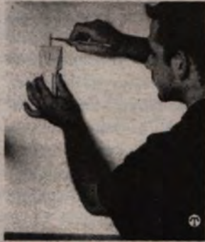
Finding the studs behind your walls is the essential first step when installing a wall safe.
