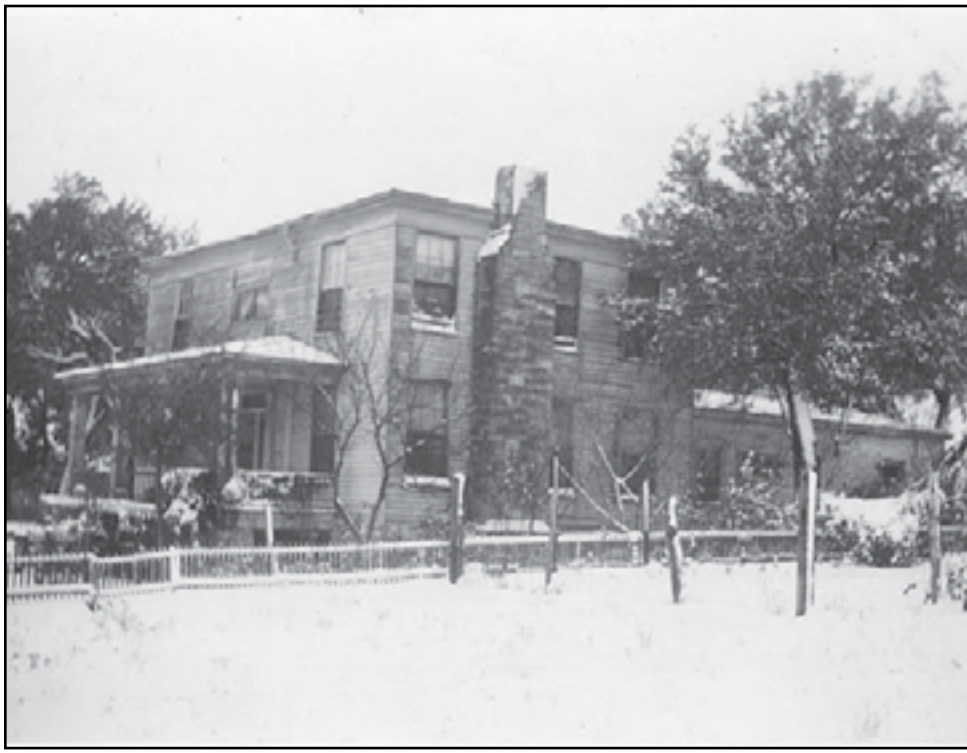
A rare shot from the North side of the house taken before it was enlarged. Although it is commonly called the Tyler House, it was built by John Thompson Flint. (SOPHIA VICKREY ARD COLLECTION)
