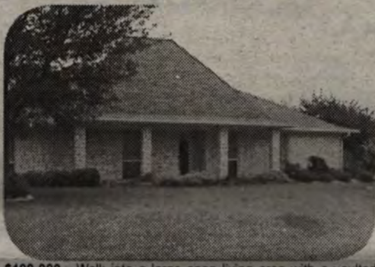
$199,000 - Walk into a large open living area with a vaulted ceiling that is enhanced with a wood burning rock fireplace. The kitchen in this home has custom made cabinets with an eat-in bar. A dining room opens into the kitchen and living area providing a wonderful place to entertain friends. A large master BR allows enough room for a sitting area or office. The other two bedrooms are separate from the master to allow for privacy.
