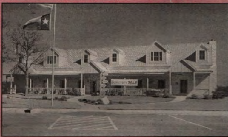
Settler's Crossing will house the Salado Public Library. Library Directors approved bids for the renovation work to begin on the Library next month. (PHOTO BY ASHLEY SMITH)
