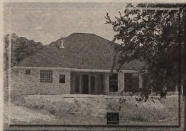
New home under construction on the golf course overlooking Salado Creek. Absolutely beautiful view. Ten to fourteen foot ceilings thruout the home. Priced at $310,000.
