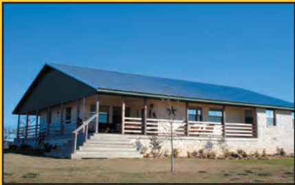
$239,900: Hilltop view of Texas countryside, private & quiet. Pier & beam construction elevates home so you can see for miles! Custom tile & backsplash in kitchen. Covered porch on two sides for relaxing with family & friends. Plenty of room for barn and horses.
