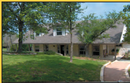
$349,500: Early Texas architecture design. 3 BR, 2.5 BA, two bonus rooms. 818 Hillcrest Dr., Salado.
