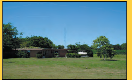
$80,000 2802 FM 2117, Temple. 6 Acres, Great Potential! House needing extensive repair, and outbuildings.
