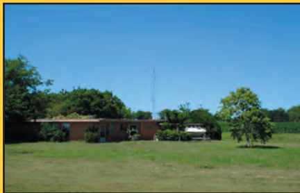
$80,000: 2802 FM 2117, Temple. 6 Acres, great potential! House needing extensive repair and outbuildings.
