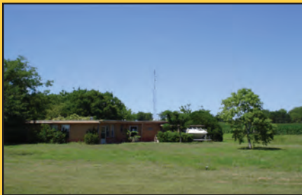
$70,000: 2802 FM 2117, Temple. 6 Acres, great potential! House needing extensive repair, and outbuildings.
