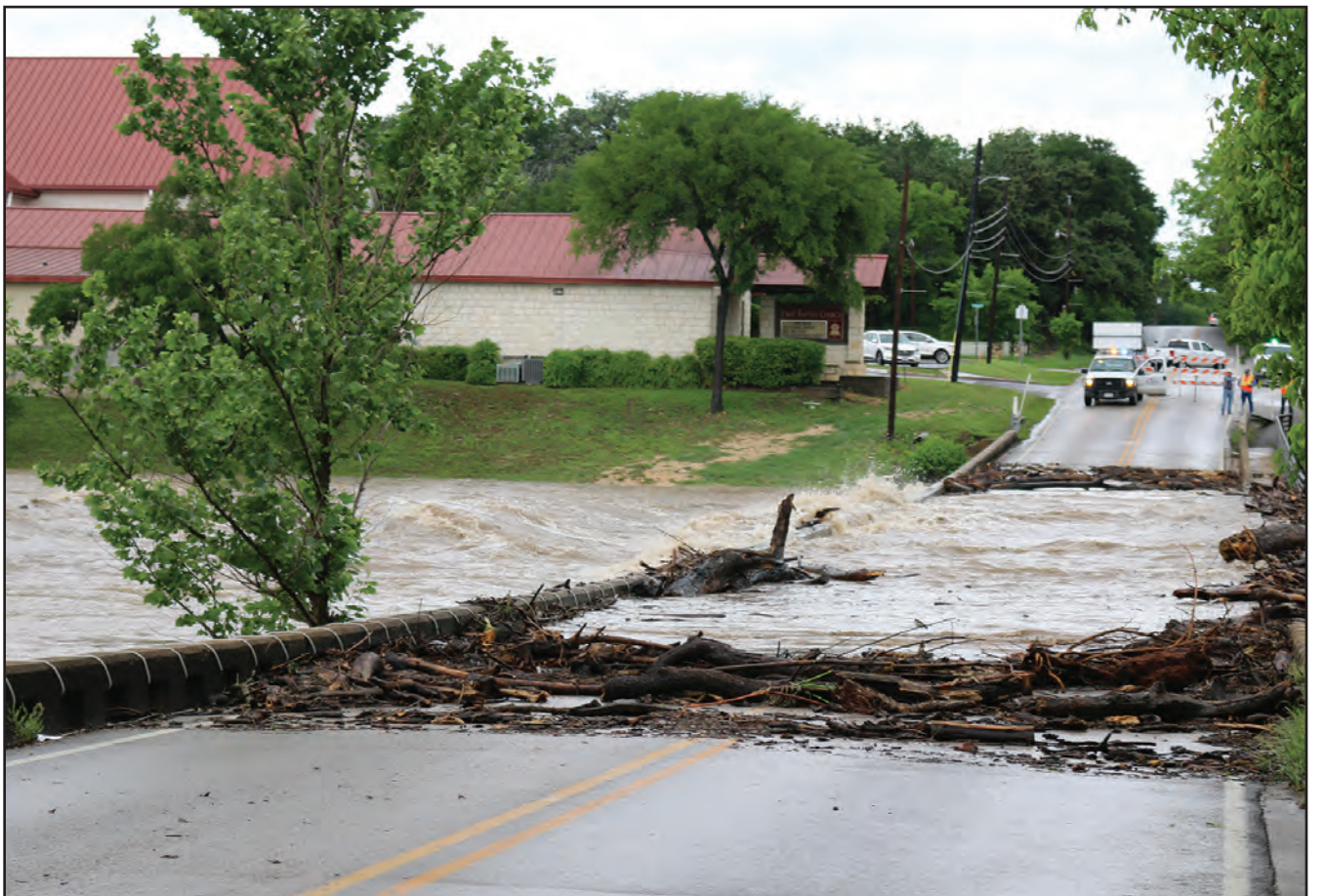
For the third time in a decade, Salado Creek flowed over the Main Street bridge after Salado received about six inches of rain overnight of May 2-3. The bridge was shut down for most of the morning on May 3 until debris could be cleaned up from it. (PHOTO BY MARILYN FLEISCHER)
