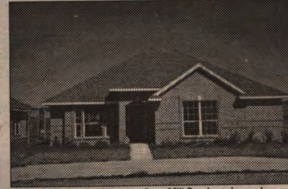
$139,900: Across the street from Mill Creek pool, pro shop and driving range. New construction. Established yard with sprinkler system. 3BR/2BA, 2 dining, large utility area. Vaulted ceiling in Master BR. Great master bath. 2+ car garage.
