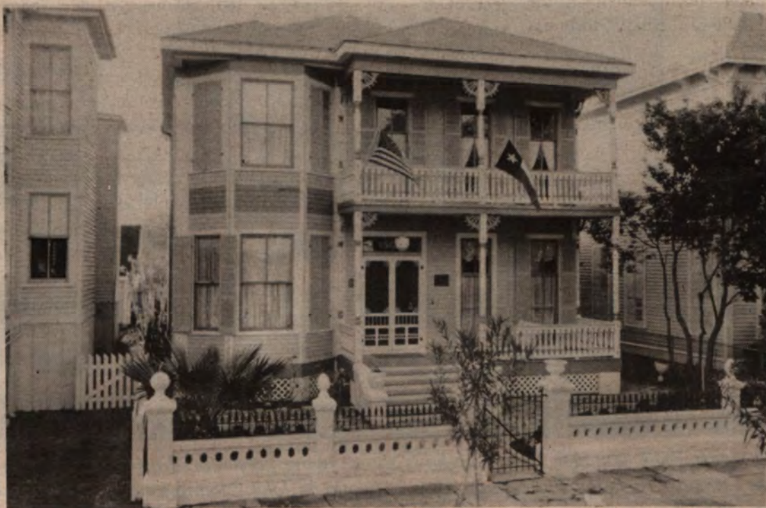
The 1890 Isaac Heffron House and nine other privately owned historic houses will be featured on the 23rd annual Galveston Historic Homes Tour May 3, 4, 10 and 11. (Photo by Bruce Bennett.)
