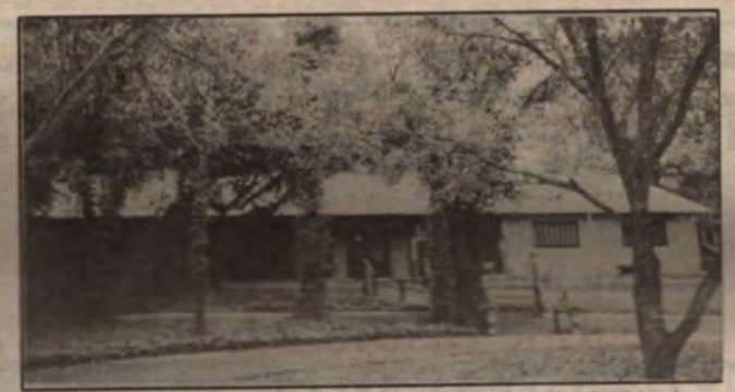
BEAUTIFUL FAMILY HOME on .868 acres at 508 South Ridge in Mill Creek. Five bedrooms, including master suite and mother-in-law quarters. Large cathedral ceiling living room with rock fireplace, built-in TV, formal dining, separate room with Jacuzzi spa. 11 ceiling fans. Totally refurbished. $189,500. Call Stew Smith.
