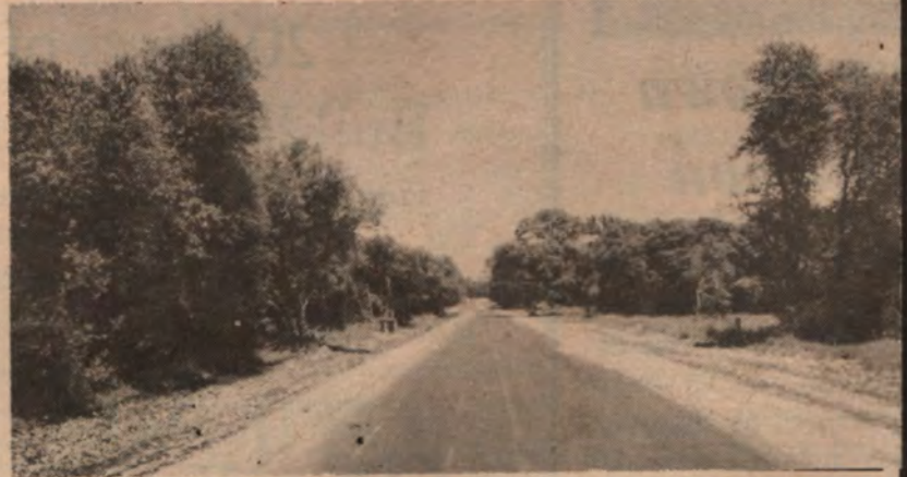
1/2 mile east of Interstate 35 on FM 2268
