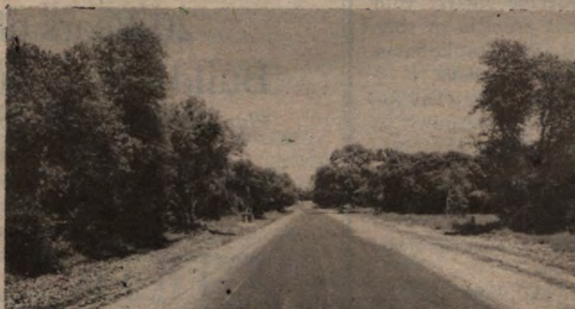
1/2 mile east of Interstate 35 on FM 2268
