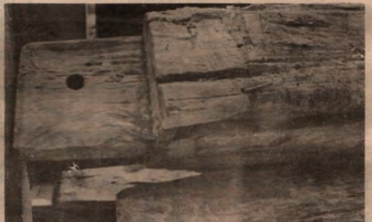
Pictured above is a detail of the hand-hewn beams from a late 19th century barn on the Winkler Farm used in decorating the new Y.O. Ranch Restaurant in Dallas' West End.
