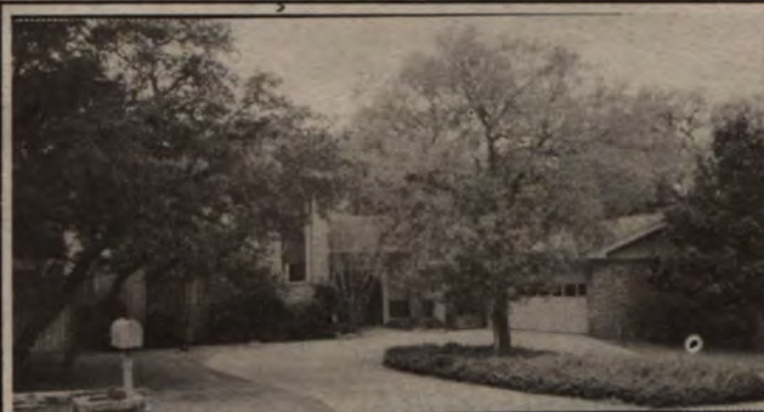
One of Mill Creek's Nicest Custom-built Homes with 4 BR, 2 living areas, 2 dining, den, office, pool and pool house, plus golf cart storage, and many more amenities! See by appointment at 1009 Arrowhead Dr. Call Stew Smith.
