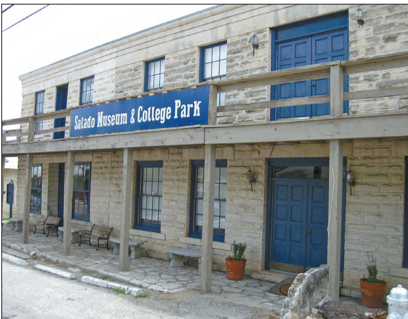
One of the final pieces in the beautification of downtown Salado will be the replacement of the balcony at Salado Museum, following the renovation of Stagecoach Inn and landscaping and sidewalk and lighting placement.
