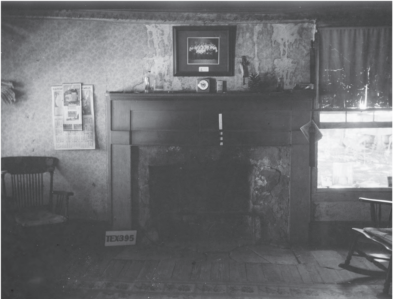
The Crockett Family once lived in the Stagecoach Inn. These photos are from 1937 and are part of the Historic American Buildings Survey.
