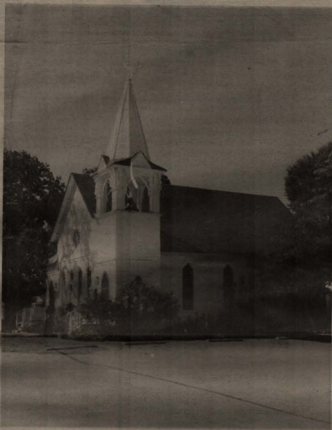
(photo by Doug Spiller) The Salado United Methodist Church, built in 1890, was restored last year and is open for tour Dec. 5-7. Tickets for the homes tour this weekend are $10 each and can be purchased at each site of the tour, as well as at the Salado Civic Center.
