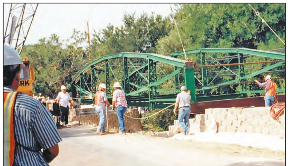
Workers guide the 87-foot bridge into place. (PHOTO BY MARY HODGE)
