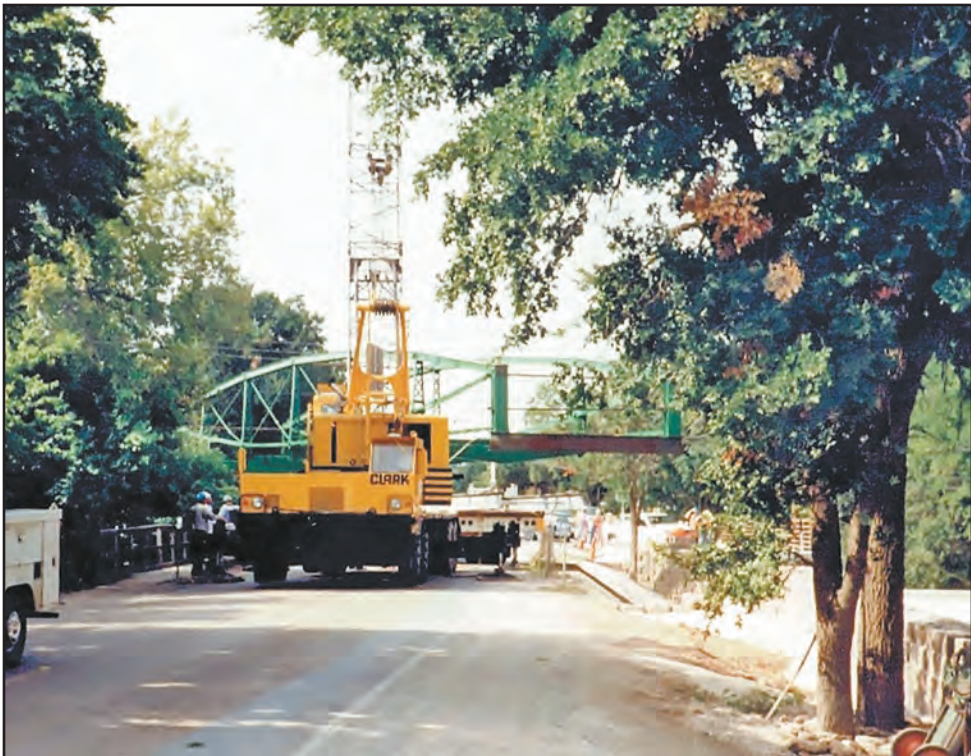
The Dodd's Creek Bridge was moved to Salado in 1997 where it spans Campbell Branch and is now a beautiful walking bridge. (PHOTO BY MARY HODGE)
