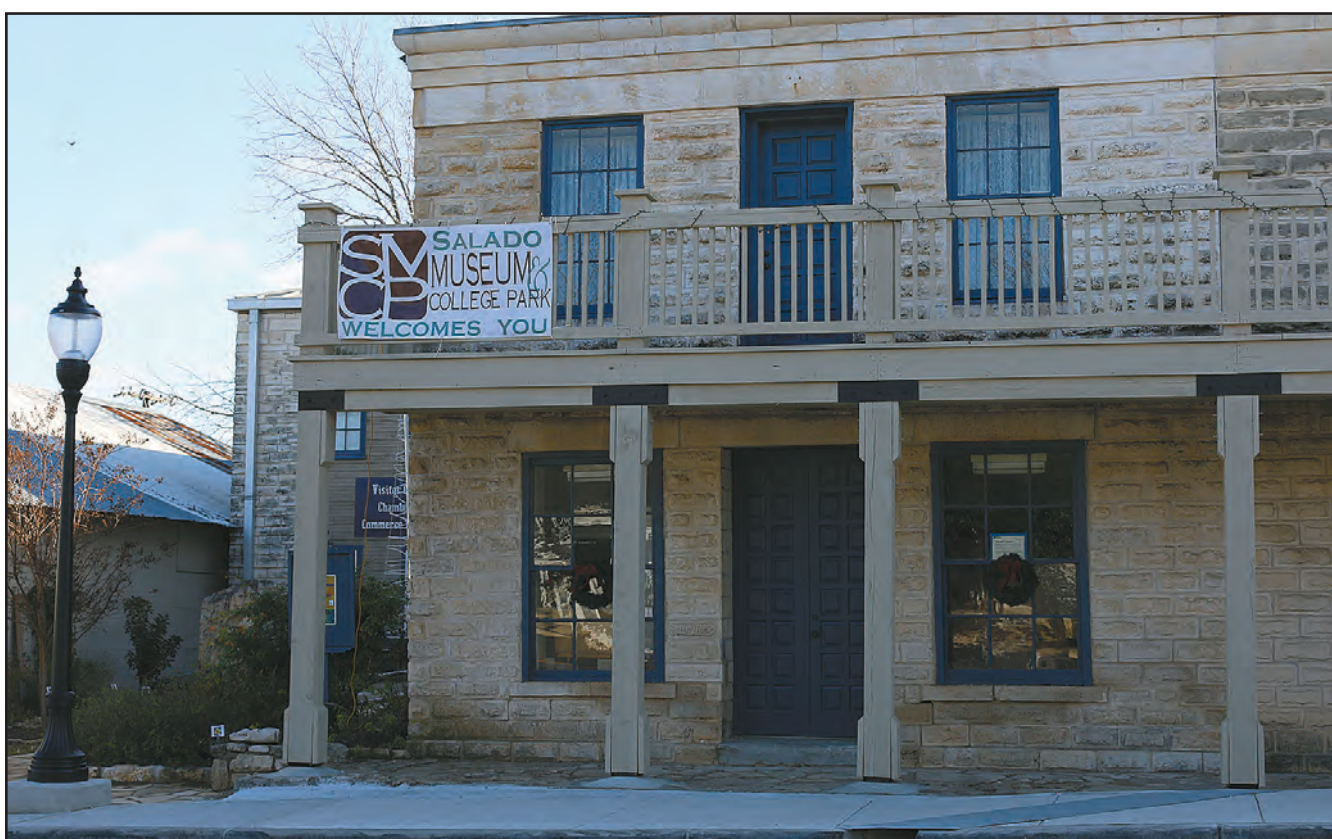
Work is complete on replacing the balcony at Salado Museum and they want you to join them in celebrating on March 13 at 6 p.m. (PHOTO BY ROYCE WIGGIN)
