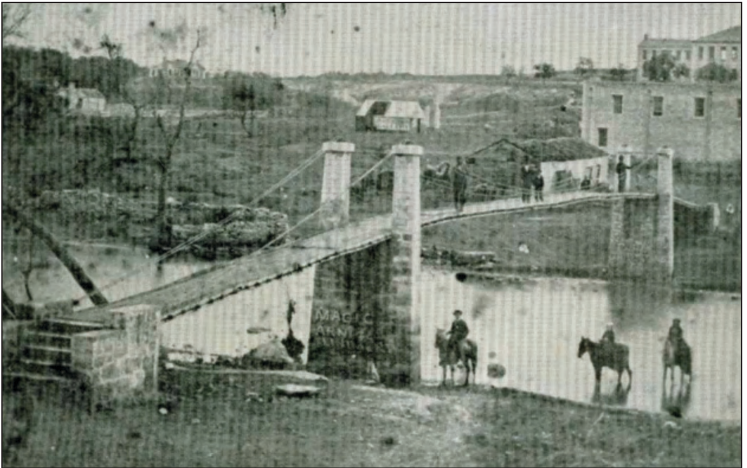
This was the first bridge across Salado Creek, built in the late 1860s.
