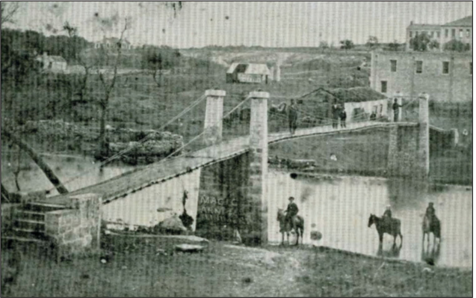
This was the first bridge across Salado Creek, built in the late 1860s.
