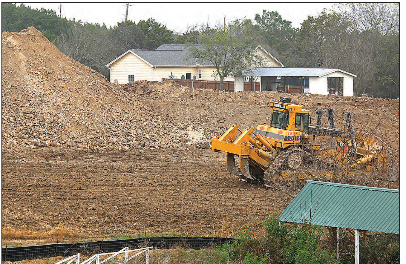
Work has begun on Water's Edge. (PHOTO BY ROYCE WIGGIN)
