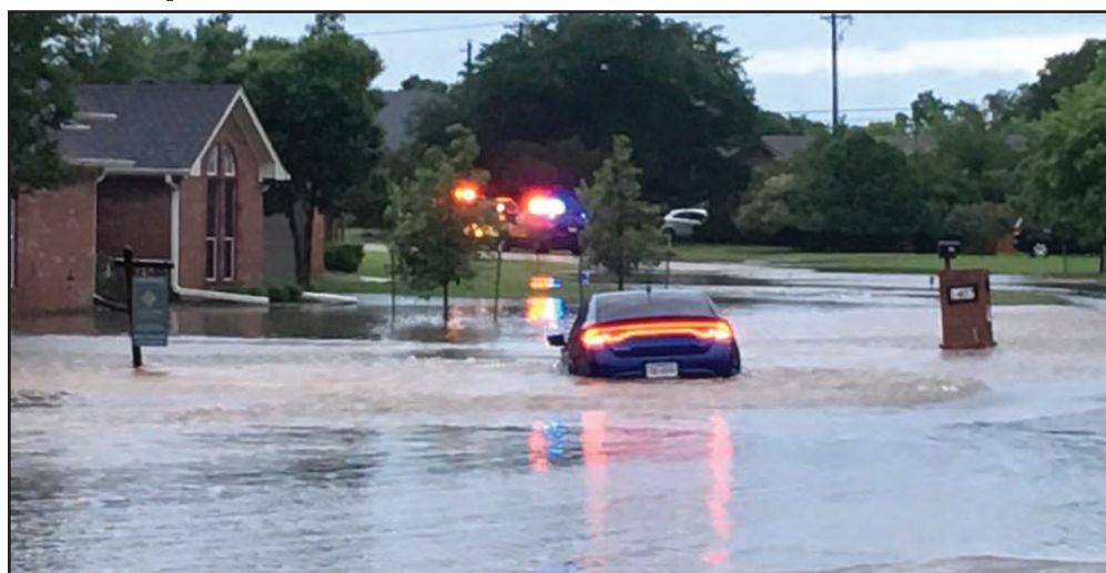
This file photo from 2019 shows a car caught in flash floodwaters on Chisholm Trail near Stagecoach Circle. The Stagecoach Circle/Chisholm Trail Improvement Project is one of the projects that the Village of Salado has submitted to U.S. Rep. John Carter's office for possible funding. (FILE PHOTO COURTESY BRUCE BOLICK)
