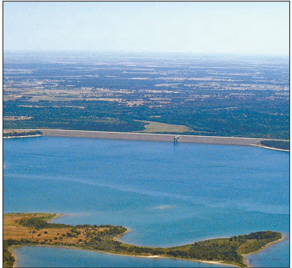
Aerial view of Stillhouse Hollow Lake and Dam on the Lampasas River in the Brazos River basin in Bell County. (U.S. Army Corps of Engineers, photographer not specified)
