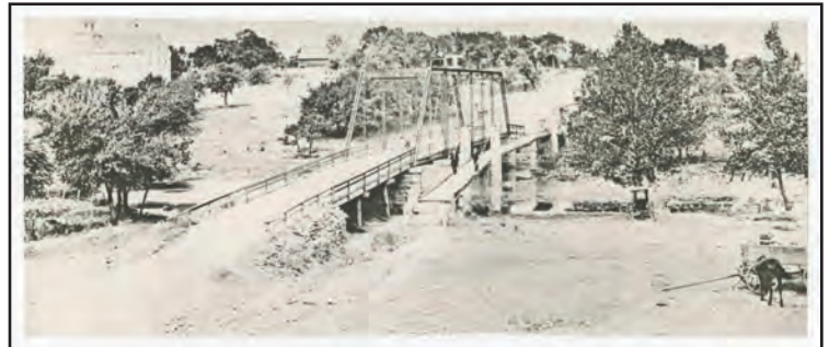
This photograph shows the first iron top wagon bridge (1892-1913) and the old foot bridge that was destroyed in 1900. (Photos courtesy Salado Historical Society)
