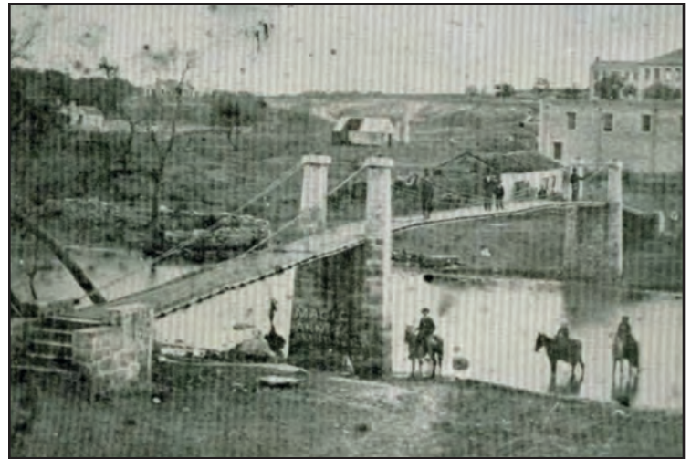
This was the first bridge across Salado Creek, built in the late 1860s.
