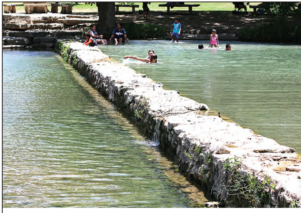
Salado Creek, fed by the springs of the Edwards A quifer, barely trickles over the low-water dam at Stagecoach Inn. (PHOTO BY ROYCE WIGGIN)
