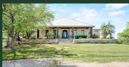
11760 Armstrong Road Beautiful large home with guest house, single level large master, separate living areas with dream kitchen and negative edge pool, shop on 146 acres with large thank hill top views. $5,995,000
